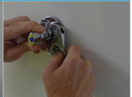
Screw on Swivel nut (with cone washer) to the threaded nipple. Then tighten with a wrench.
