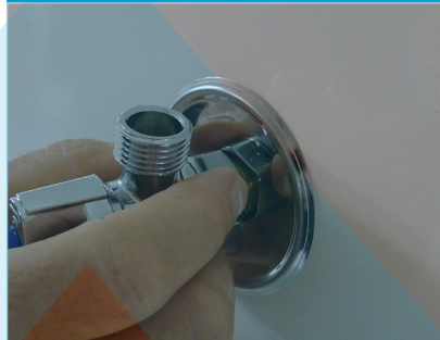
Align stop outlet to the correct position
