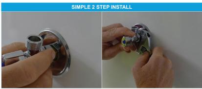
Align stop outlet to the correct position
