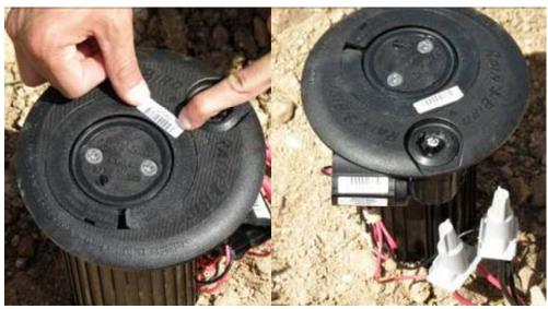
In addition, the label can be scanned prior to the rotor being backfilled using a Rain Bird scanner.
