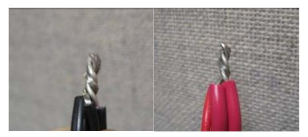
Use Rain Bird DB splice kits to ensure waterproof splices and provide strain relief. Trim the twisted bare ends of the wires to 5/8" (15.9 mm) in length before inserting in the DB splice kit. The DB splice kit has a wire length gauge on the underside of the flange to assure proper wire length.
